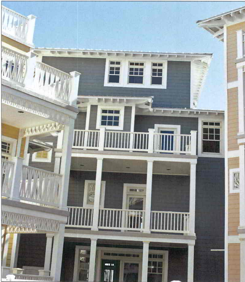
Rear Elevation Looking at Pool
