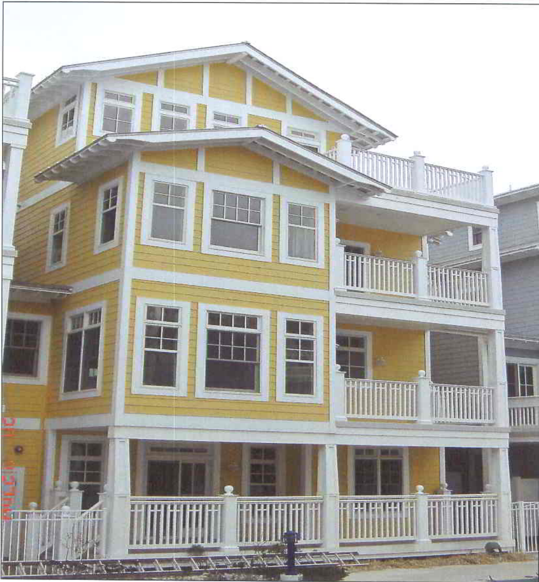
North Elevation at Pool
