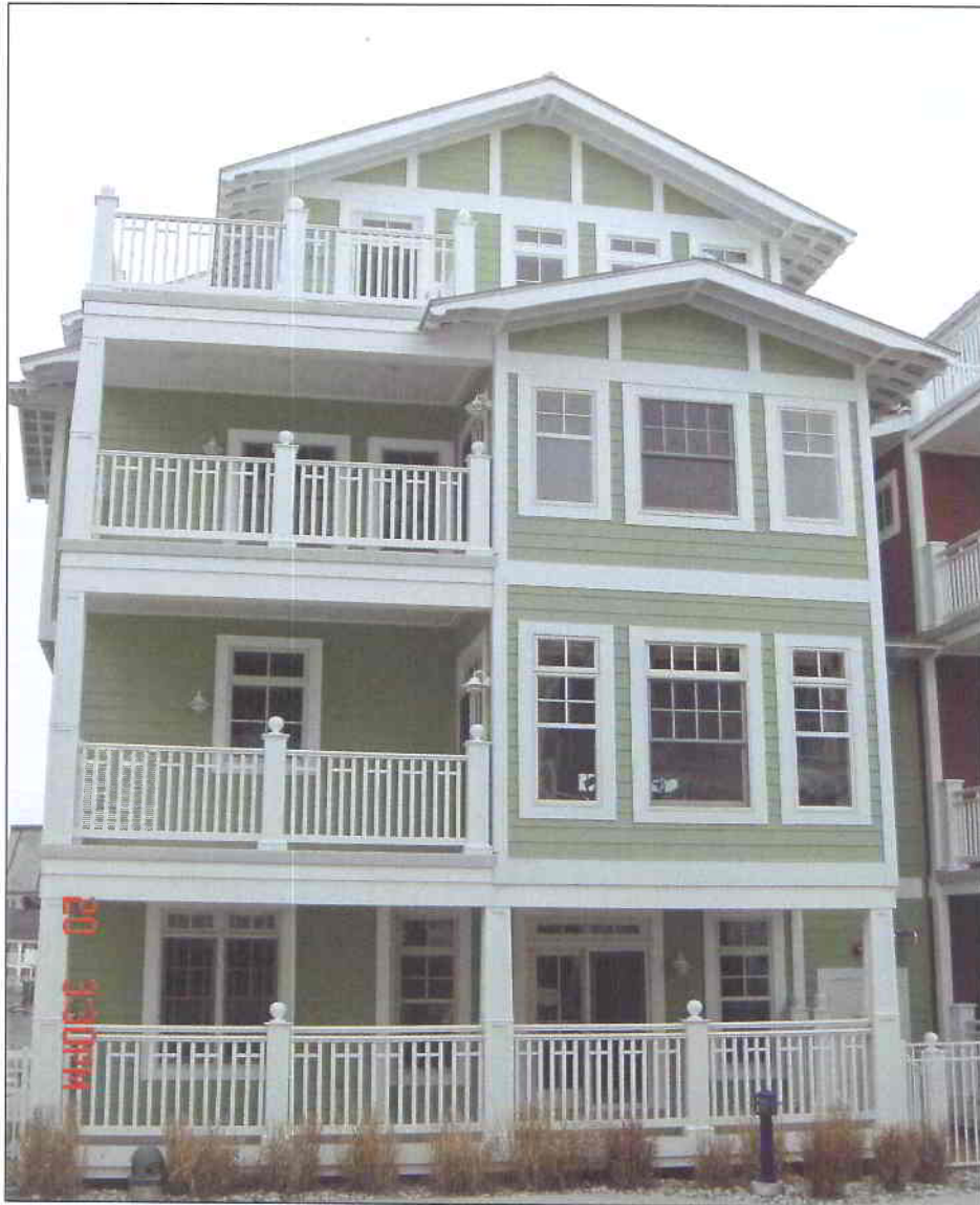
South Elevation at Pool
