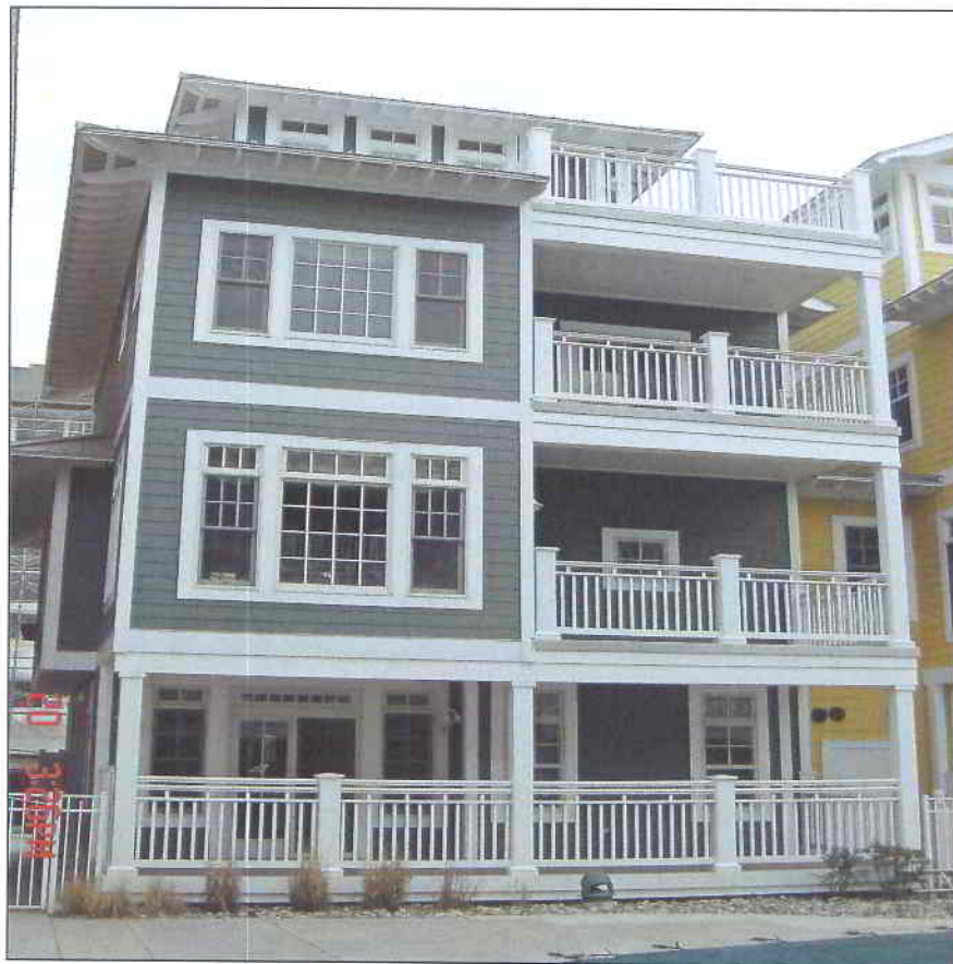
North Elevation at Pool
